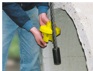
Drop pipe carrier lifting sling through hole in pipe. Align and insert "Tea Cup" pipe carrier into lifting sling.
